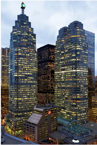
Brookfield Place Bay Wellington Tower
