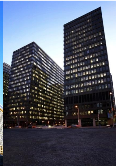
Jean Edmonds Towers (two buildings)
